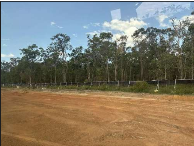
Photo Set 2: Temporary koala exclusion fencing adjacent to clearing activities and retained corridor.
